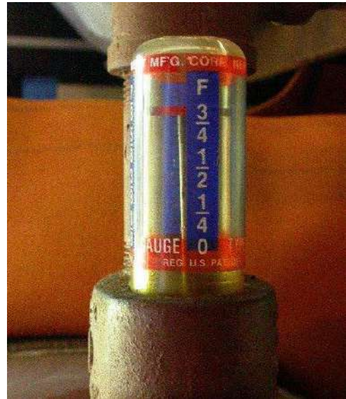
A U.S. patented float type fuel level indicator on top of a cylindrical horizontal tank showing “FULL”, “3/4”, “1/2”, “1/4” and “0 or EMPTY”.
